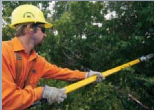
Ensuring trees are not growing too close to power lines
