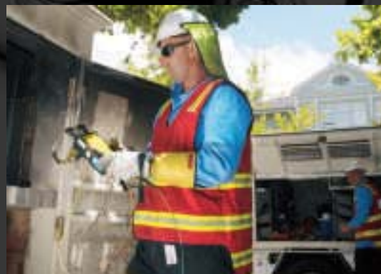
Installing an interval meter in Melbourne's inner suburbs
