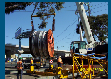
Loading the cable on to the cable stands
